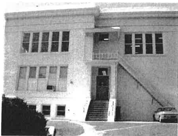
Photo 8.3: Southside elevation. View shows the multiple levels of the building.
