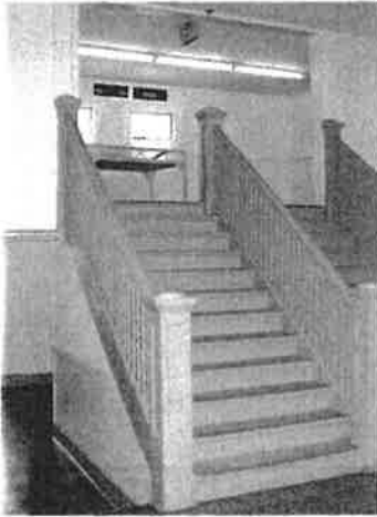
Photo 3.1: Main Stair at the front entry. It also steps down to the left of the stair. The landing seen in this photo is only about half way up to the 2 nd floor level.
