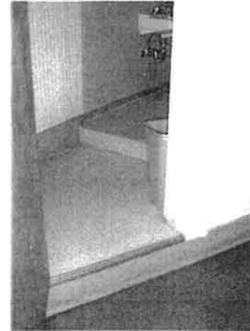
Photo3.3: Hallway to restroom change in levels.
