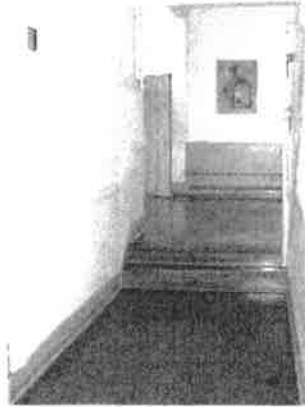
Photo3.2: Change in level at the hallway on the 1 st floor level.
