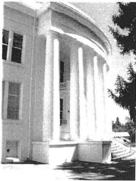
Photo 8.1: Front entry from the north. Notice the window mounted air-conditioning unit in the lower window at the porch.
