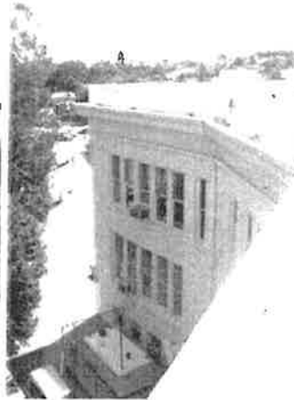
Photo 5.2: Window mounted air-conditioning units on the back side of the building.
